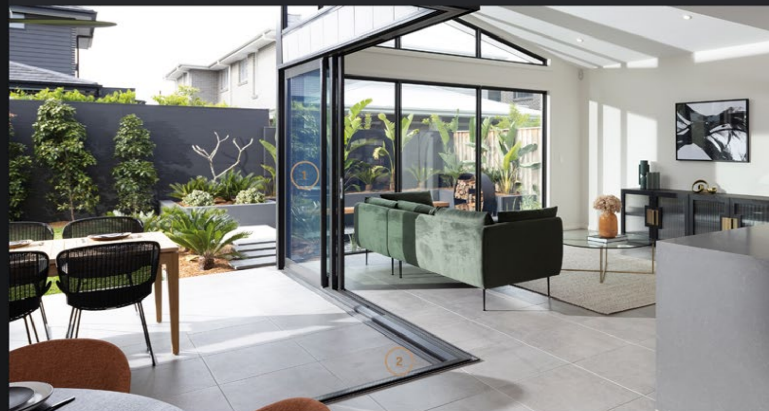
2410mm Increased Door Height & Recessed Slab for Flush Tracks to Stacker Doors
